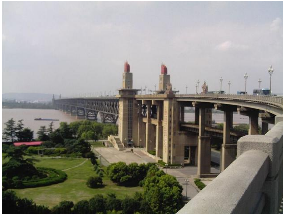
Nanjing Yangtze River Bridge in Jiangsu Province
