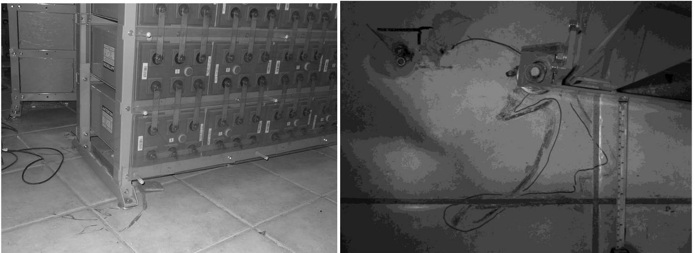
*Fig. 8a. (left) Rack of batteries that was moved across the floor during the mainshock. The near (short) edge of the front rack is aligned roughly N-S, with the closest edge towards the south. 8b (right) close-up of scratches left on tile, including pen marks drawn to indicate inferred trajectory. (The loop is inferred to have been left by a remnant of the bolt that was dragged as the rack moved)*
