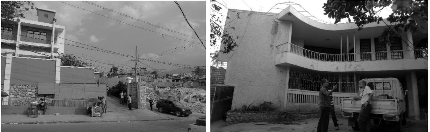
Figure 5a (left) A good-quality commercial structure in which MMI V-VI is estimated based on an eyewitness interview; 5b (right) a private home, masonry C construction, for which MMI VI is estimated. The structures on both sides of the structure shown in 5a collapsed catastrophically, as did a school building adjacent to the house shown in 5b.
