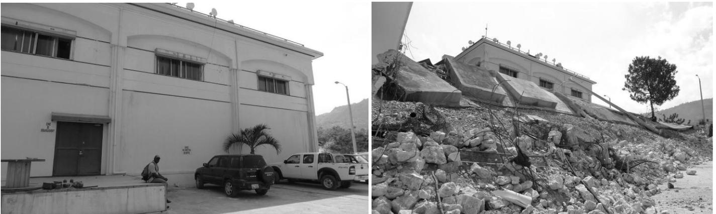
Figure 6a. (left) Canape Vert Voila cell phone facility; 6b. (right) collapse of retaining wall in parking lot. The face of the building seen in the photograph is aligned roughly N-S; the battery racks discussed in this study are located on the ground floor, in a large room behind the doors seen at left in Fig. 6a.
