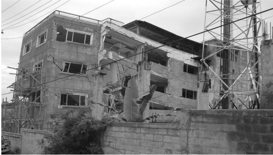
*Figure 7. Damage to recently built commercial building approximately 0.5 kilometer west of HVCV. The building was later demolished.*
